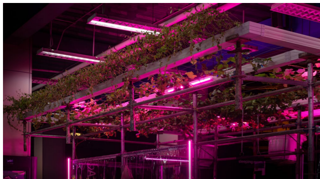
gutter as a device for plants holder and the installation's electrical system
