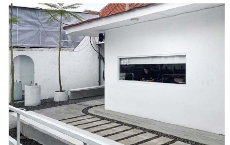
one of tenant's facade
