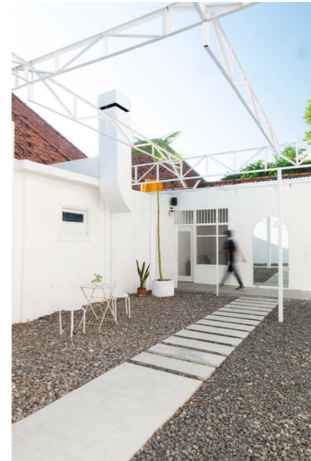
the existing struss above are preserved and designed to become supporting rigging system for exhibition, music performance, or movie screening
