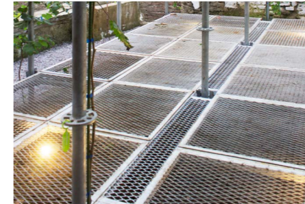
expanded metal allows natural light and airflow to go through to the soil while still able to functioned as a rigid platform
