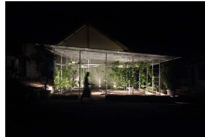
the front side of the building
